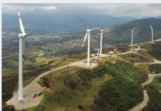
Villonaco wind farm in Ecuador 55
