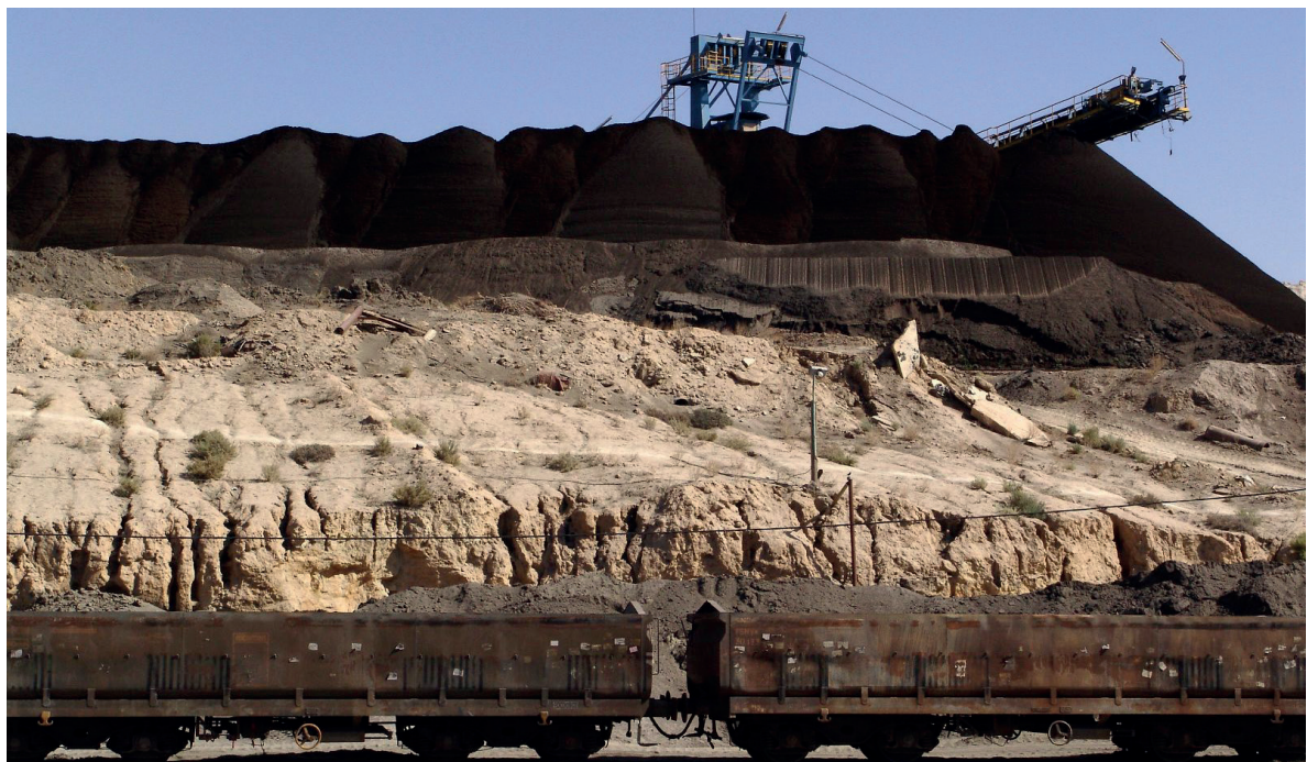
Railway station at Seldja potassium plant
